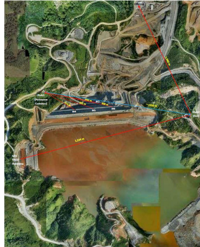
DT Datalogger and RSTAR Telemetry
