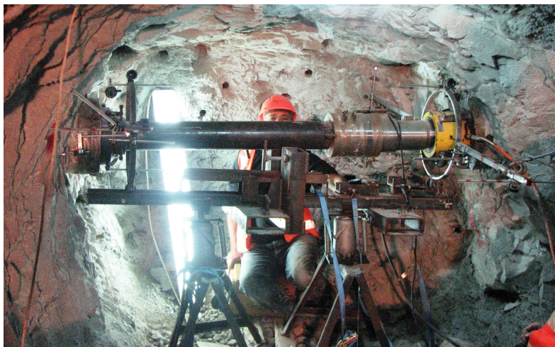
Fig. 6: Horizontal setting of the Plate Loading Test. (Performed by the Building and Infrastructure Testing Lab. Israel)
