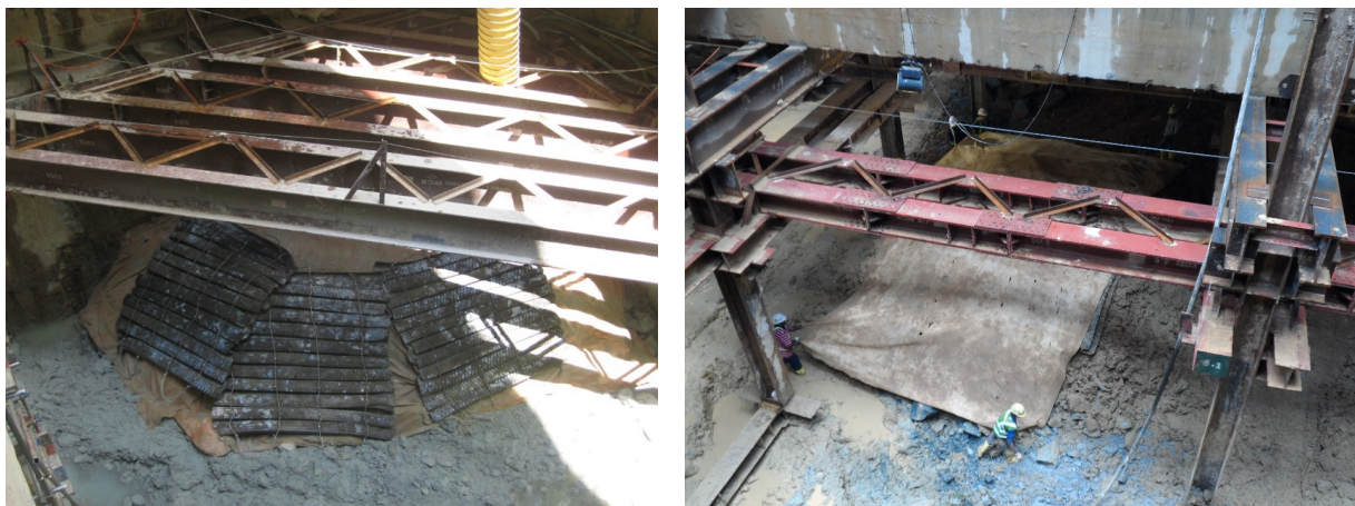
Fig.9. Overburden backfilling at blasting area
