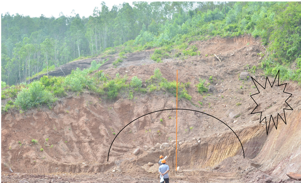
Fig. 1 South portal of North tunnel, fault zone grade V, right side main view from South portal;
