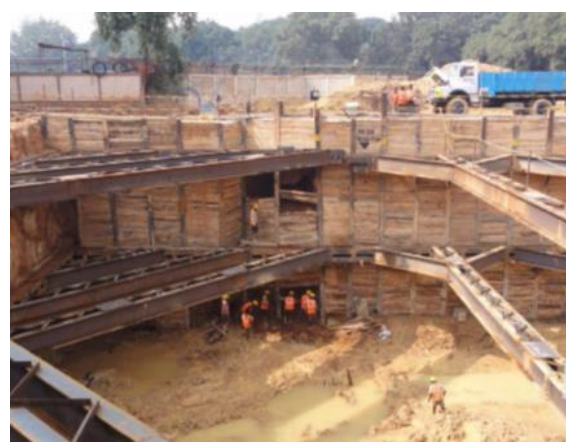
Fig. 3. Loss of soil behind the wall at Cricket stadium
