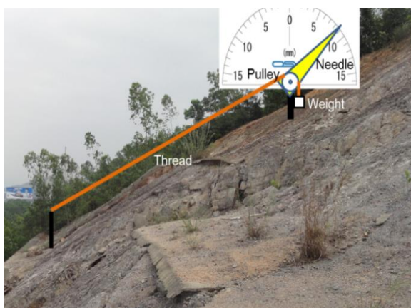
Fig. 6. Monitoring image: Mechanical displacement sensor
