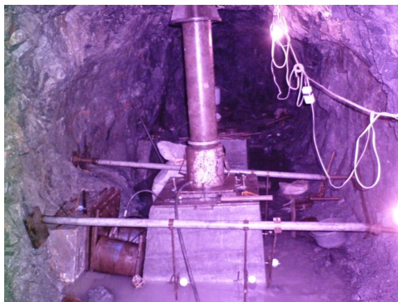
Fig.3a: typical test arrangement
