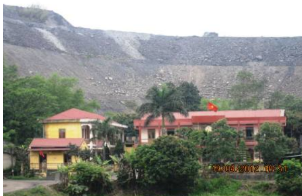
Fig. 1a. Civil works at waste dump's food
