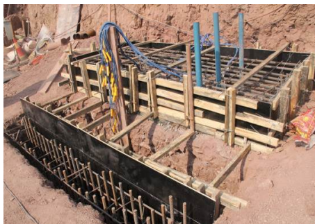
Fig. 4. Site layout of micropiles composite structure.
