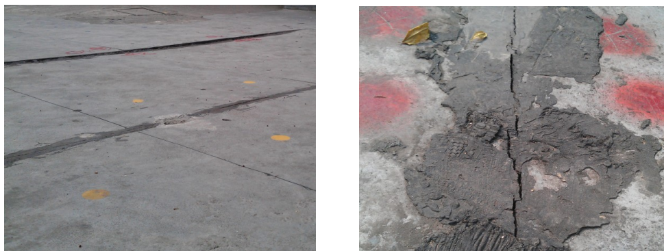
Fig.7. Photos of surface tensile cracks
